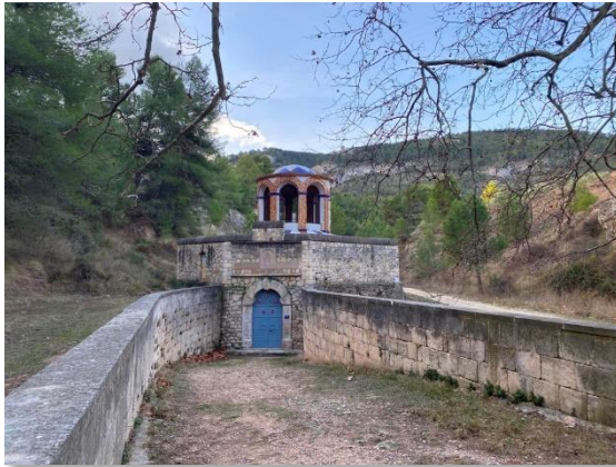
Figura 5. Vista exterior Manantial Molinar
